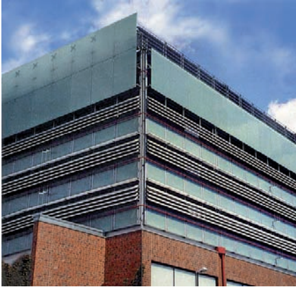
▲ Office complex. Horizontally mounted c|sairfoil® blades AF 320 LB provide effective sun control, reduce considerably noise from the outside getting into the building and integrate stylishly with the architecture of the glass facade.
