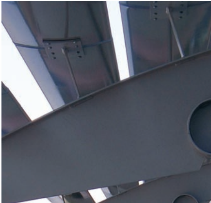
▲ Custom blade supports. The custom blade supports shown have been specifically designed for cantilevered projections of Audi showrooms. c|sairfoil AF270 blades are fixed onto vertical custom-made supports, attached to horizontal support segments. The lightweight but extremely robust structure of c|sairfoil blades allow for the design of any imaginable support, fixture, suspension or attachment, proofing to be an extremely versatile, architectural design element and sun control system at the same time.
